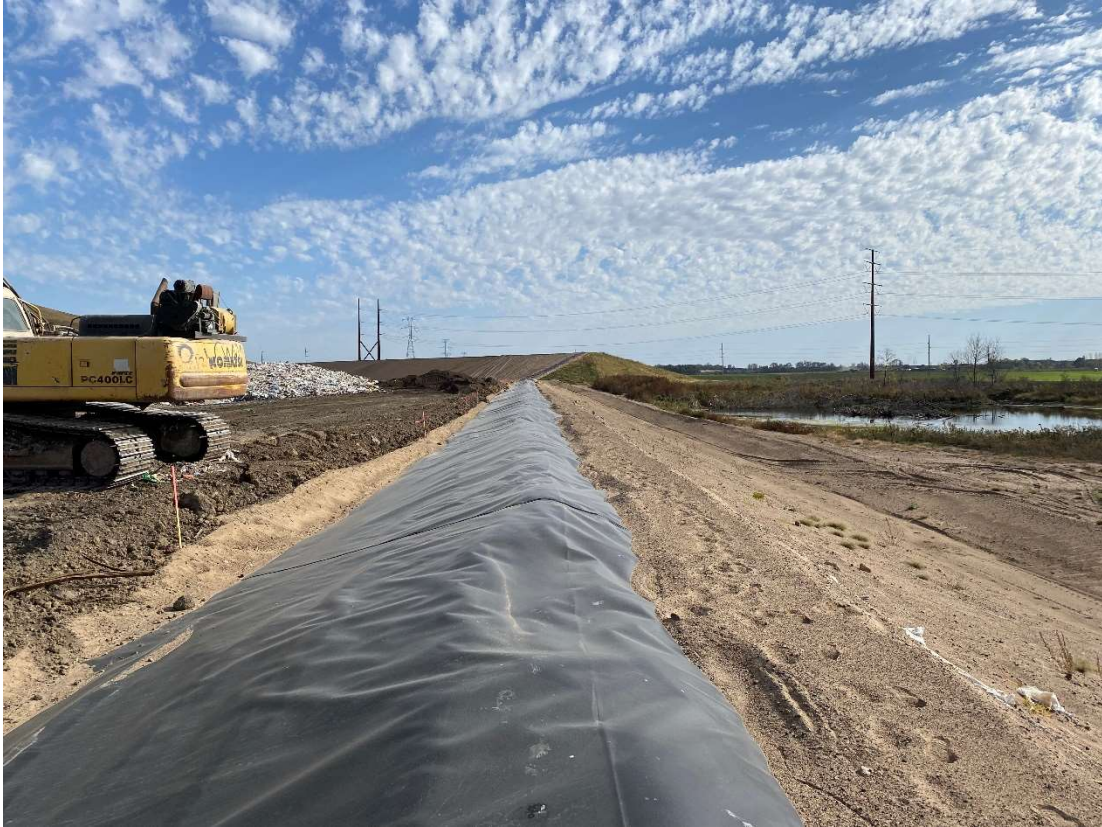
Location 11 – Cell 6, SW corner, looking southeast
