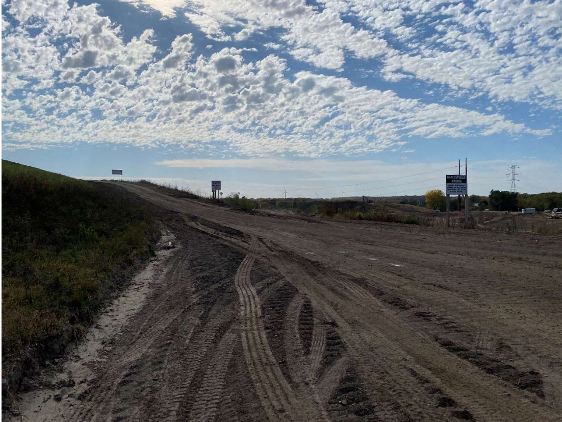
Location 14 – Looking Southwest, Cell 2A Northwestern Waste Slope and Anchor Trench
