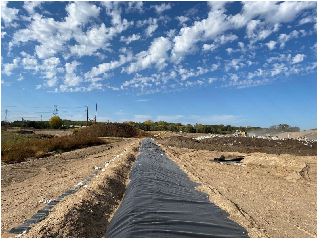
Location 10 – Cell 6, SW limit at midpoint, looking northwest
