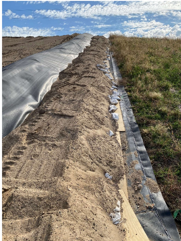
Location 9 – Cell 6, looking south
