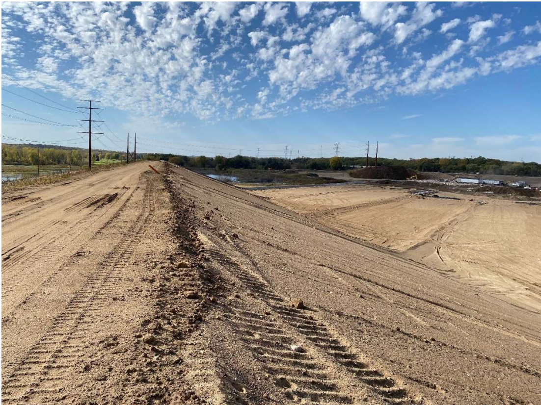
Location 7 – Cell 6, midpoint of inner berm, looking west
