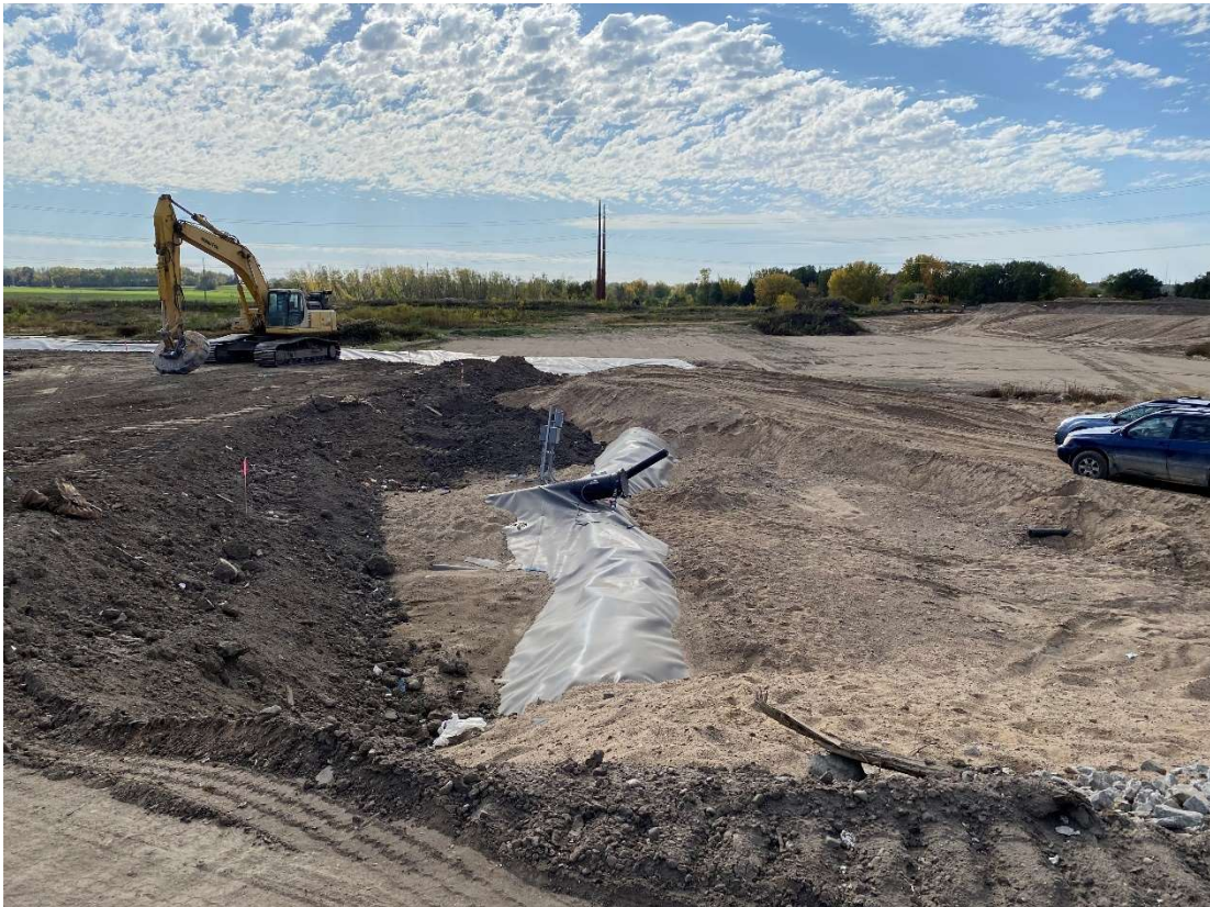
Location 12 – Cell 6, midpoint of NW limit, looking southwest
