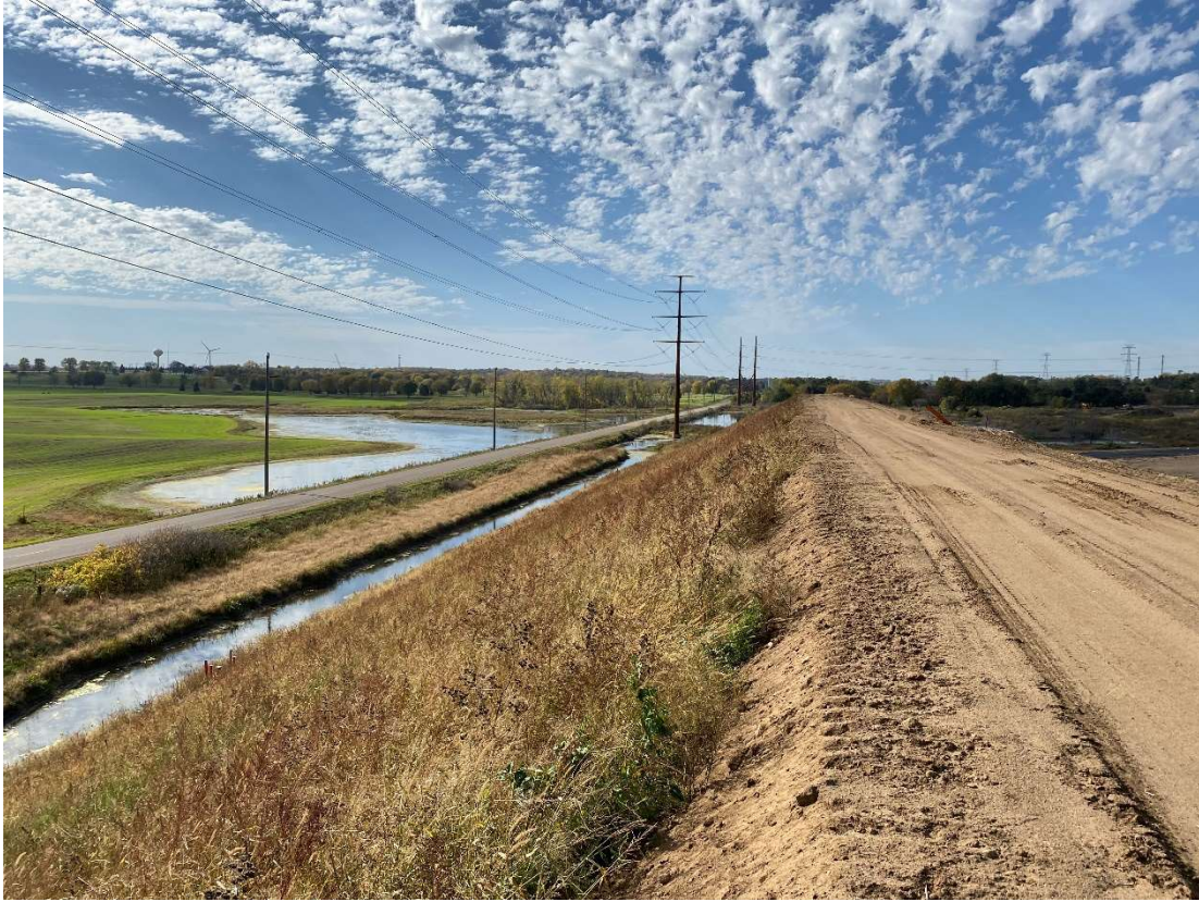
Location 7 – Cell 6, midpoint of outer berm, looking west
