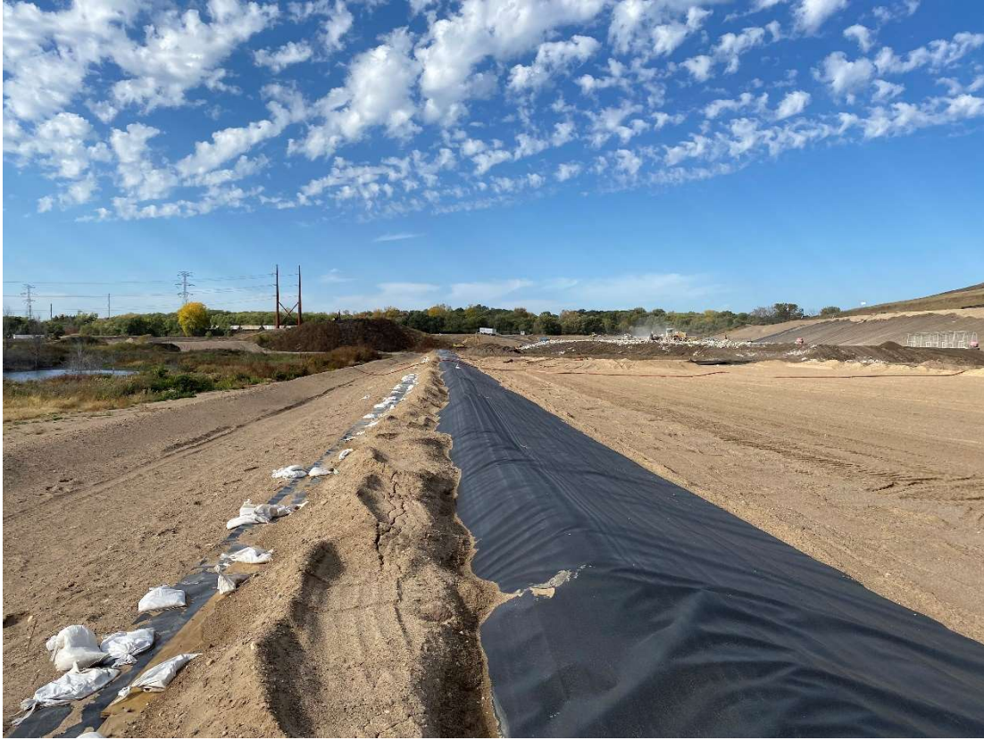
Location 9 – Cell 6, looking northwest
