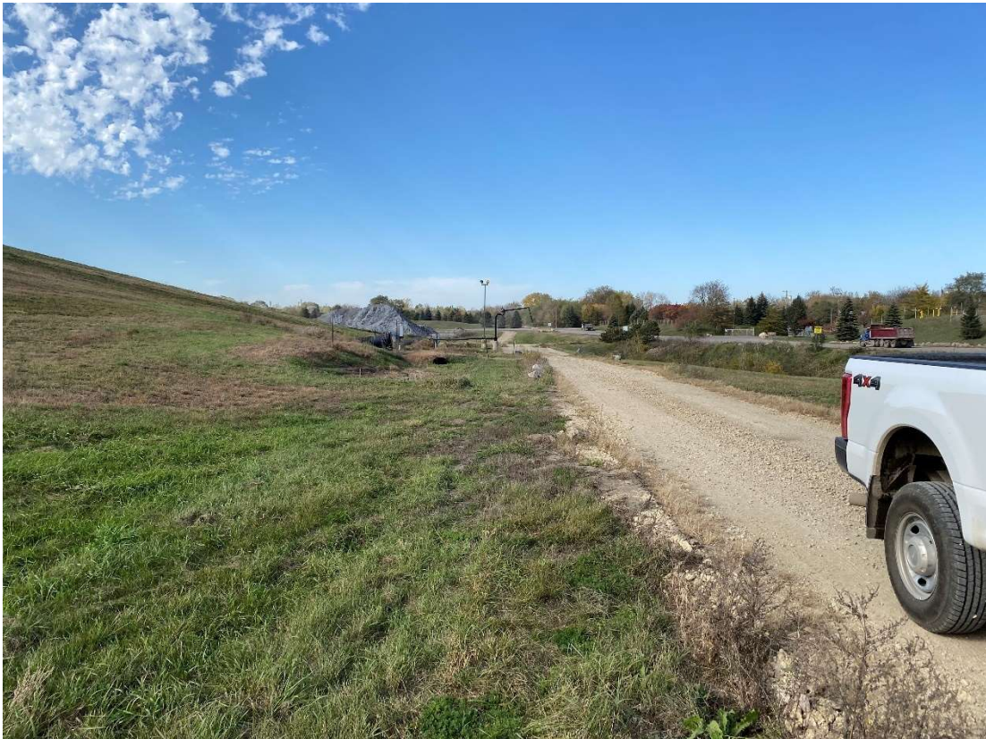
Location 1 – Looking Northwest, Cell 3 Berm
