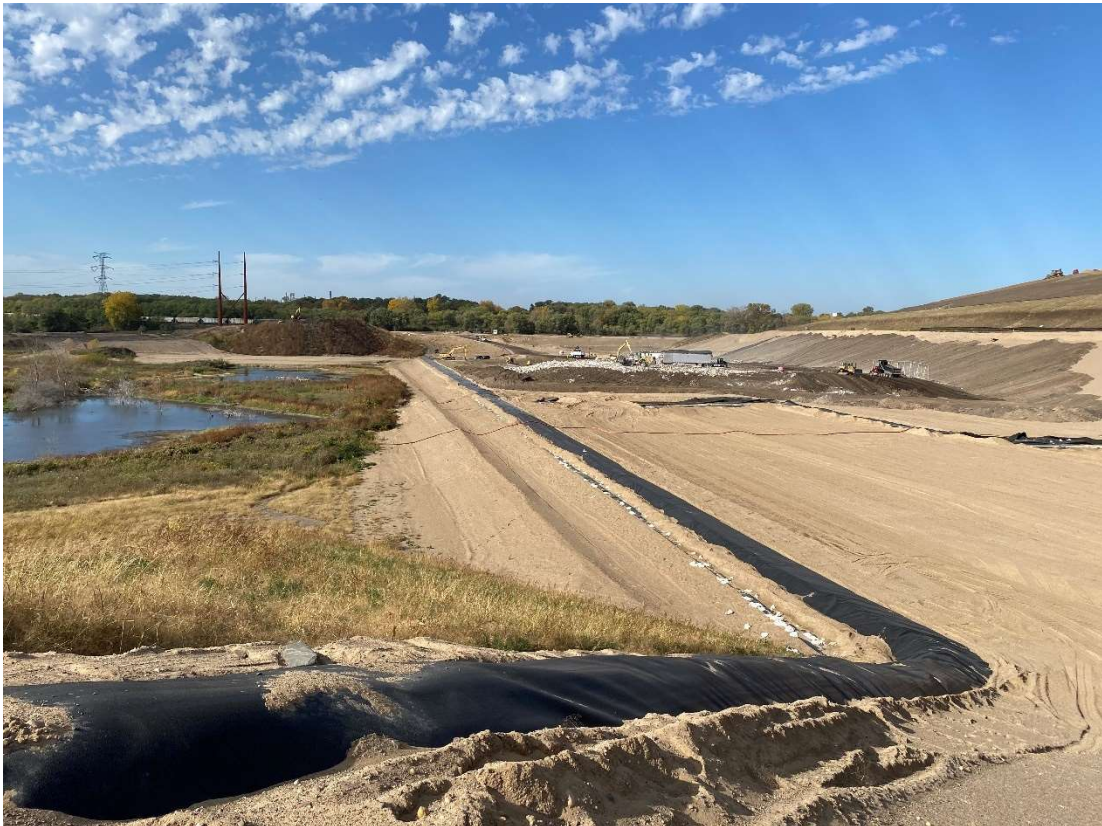
Location 8 – Cell 6, SW corner inner berm, looking west
