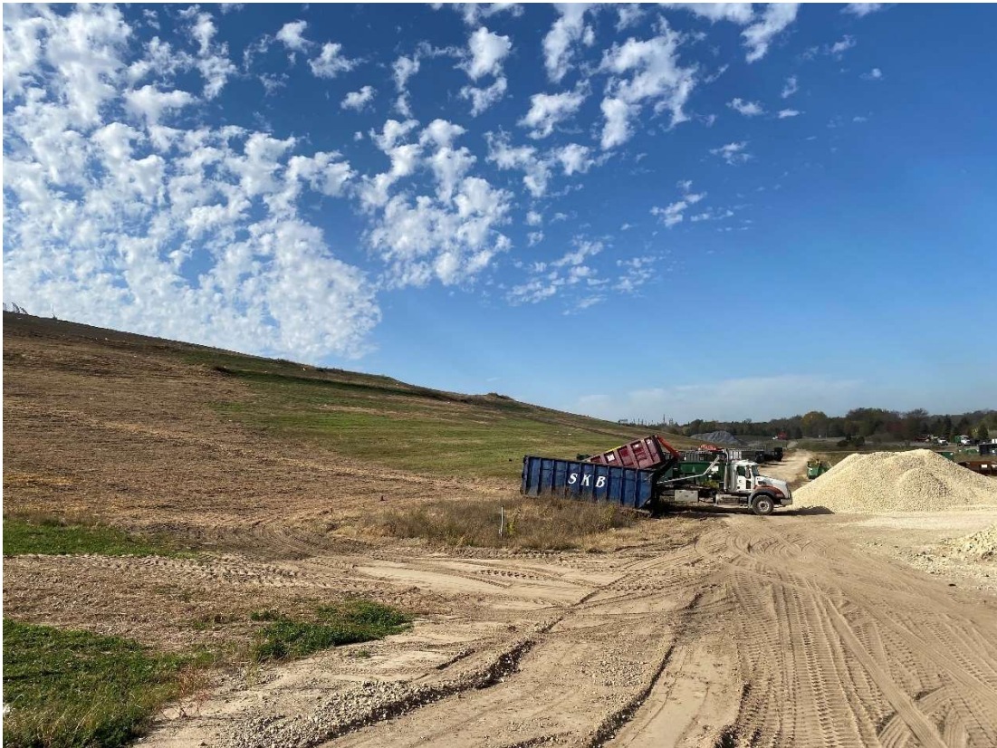
Location 3 – Looking Northwest, Phase 3A Anchor Trench and Northeastern Waste Slope
