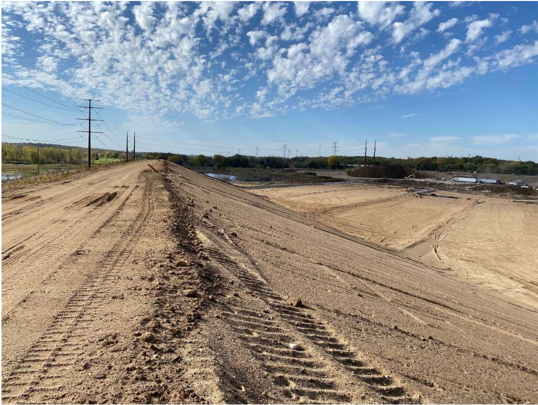
Location 6 – Cell 6 SE corner, inner berm, looking west
