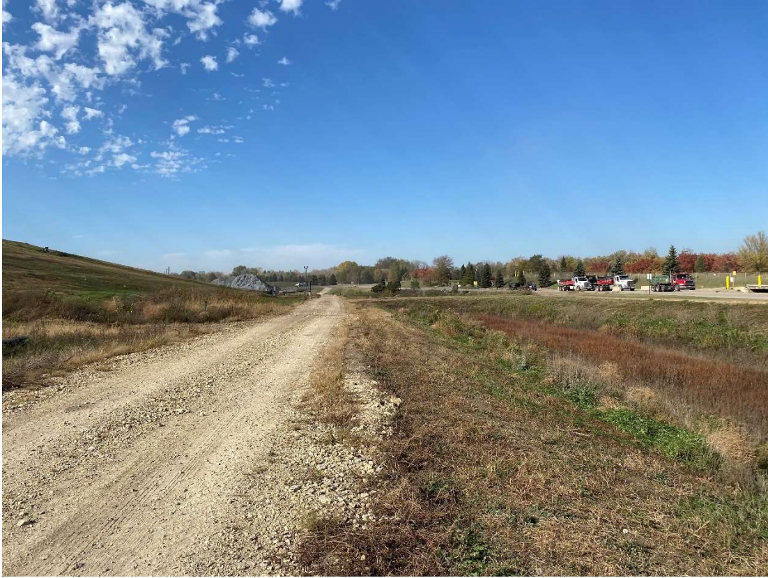
Location 2 – Looking Northwest, Cell 3 Berm & Stormwater Pond
