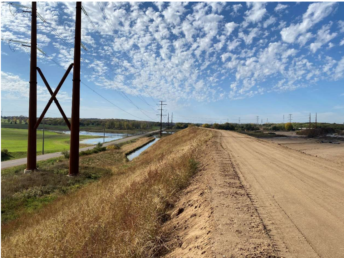
Location 6 – Cell 6 SE corner, outer berm, looking west
