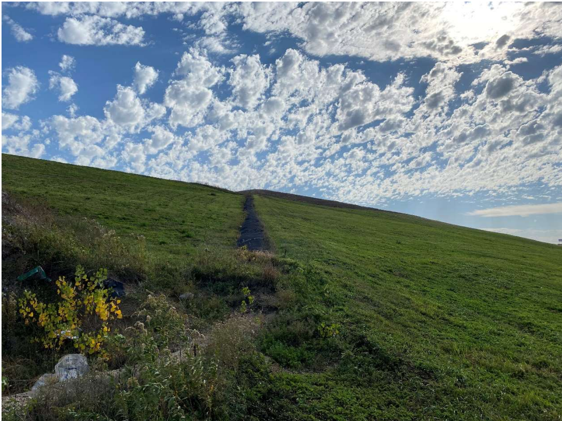
Location 15 – Looking South, Edge of Cap over Cell 1
