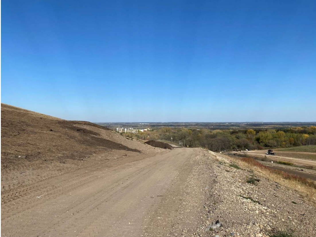
Location 4 – Looking Northeast, Phase 3 Liner Limit
