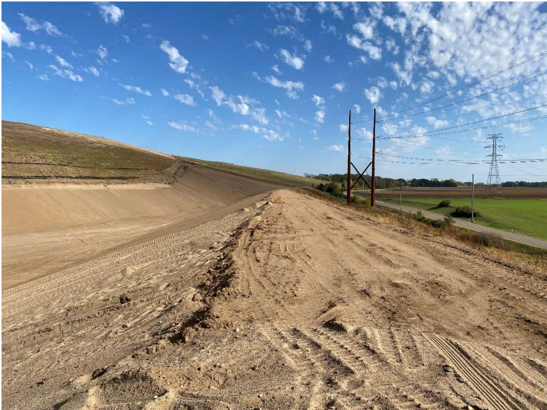
Location 8 – Cell 6, SW corner inner berm, looking east
