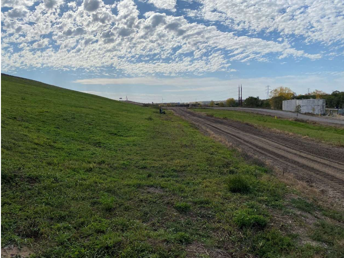
Location 15 – Looking Southwest, Cell 1 Toe of Waste Slope
