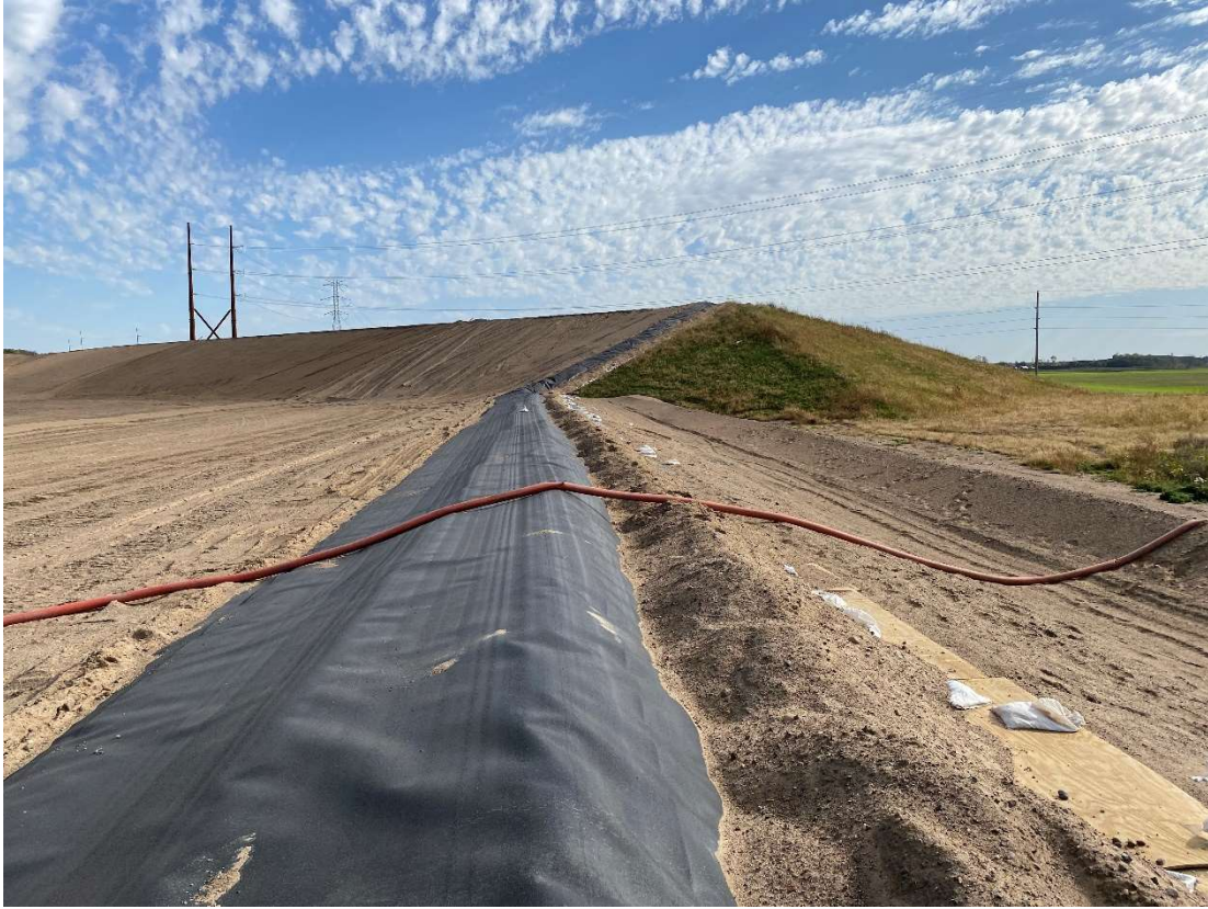
Location 10 – Cell 6, SW limit at midpoint, looking southeast
