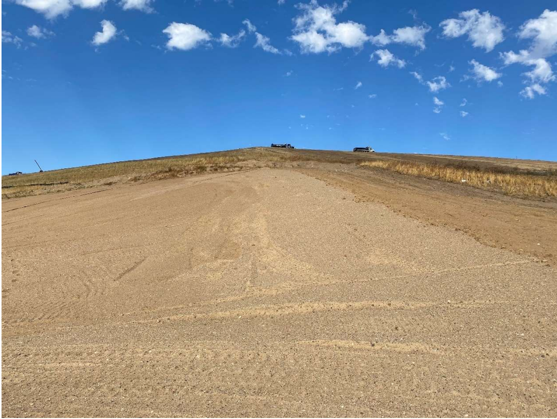
Location 6 – Cell 6, SE corner Looking northwest
