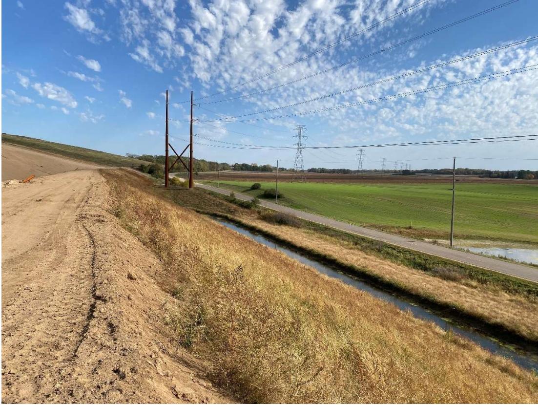
Location 8 – Cell 6, SW corner outer berm, looking east
