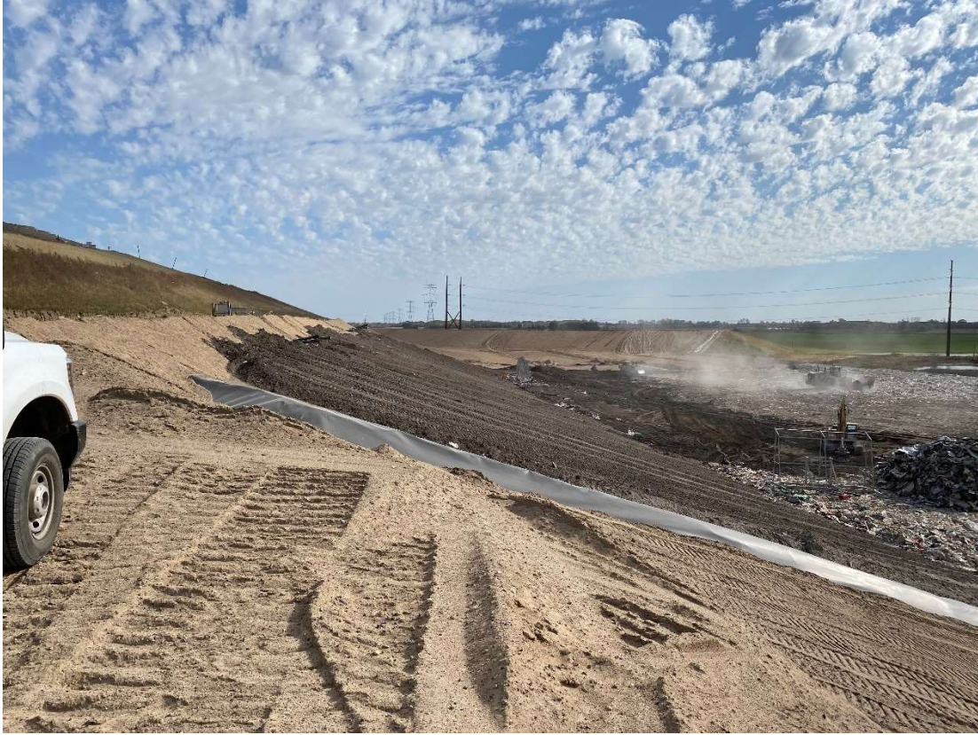
Location 13 – Looking Southeast, Cell 2A Southwestern Berm and into Cell 6
