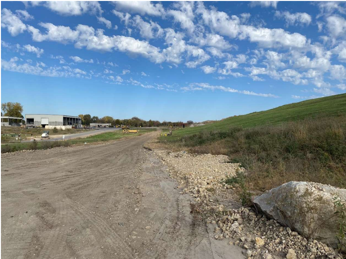
Location 14 – Looking Northeast, Cell 1 Northwestern Waste Slope
