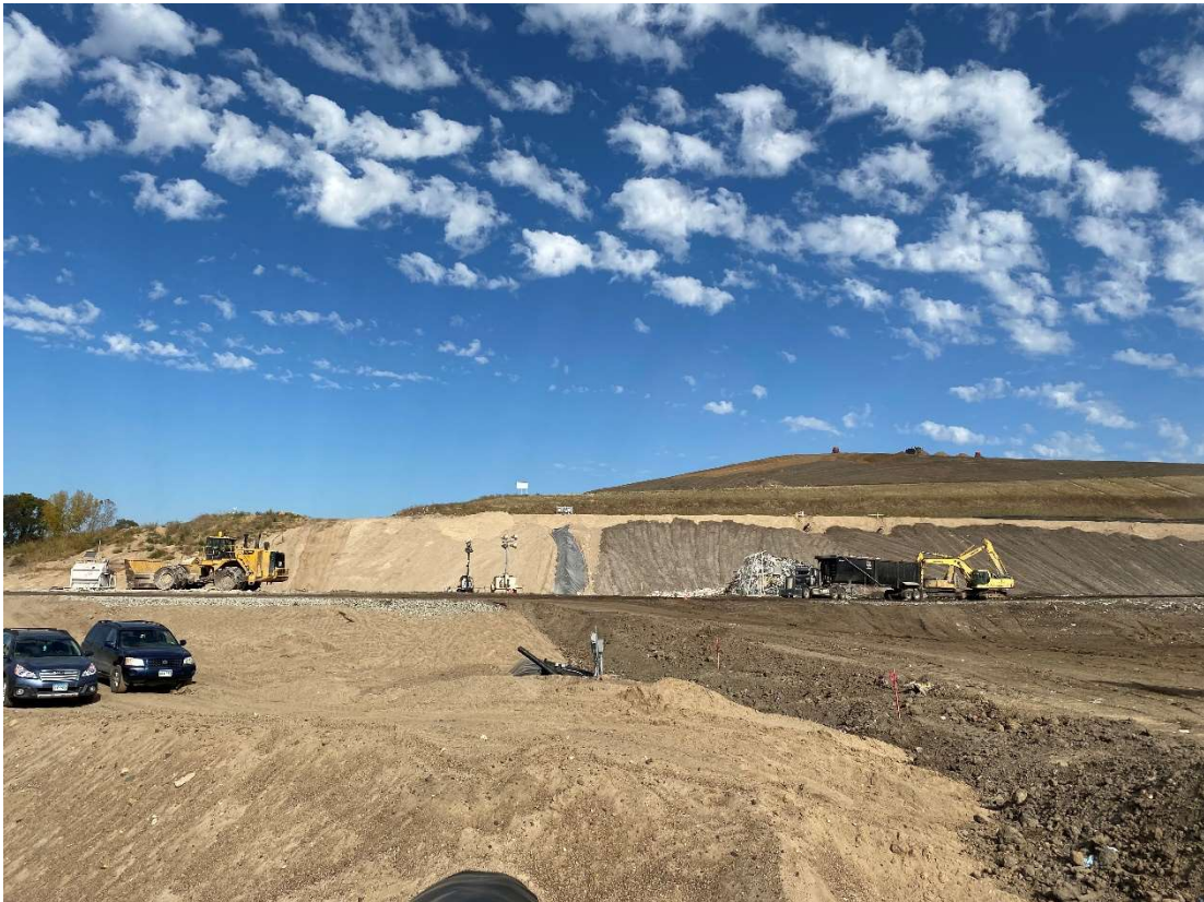
Location 11 – Cell 6, SW corner, looking northeast
