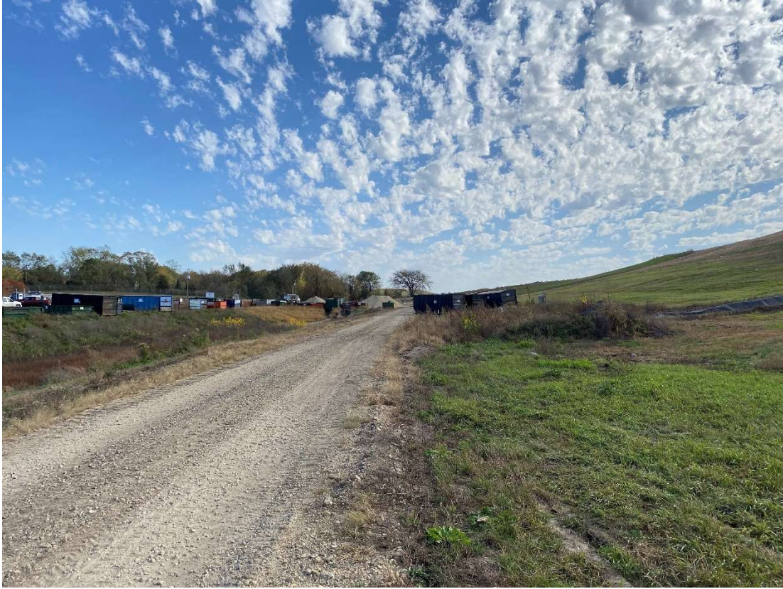
Location 1 – Looking Southeast, Cell 3A & 3B Waste Slope & Anchor Trench
